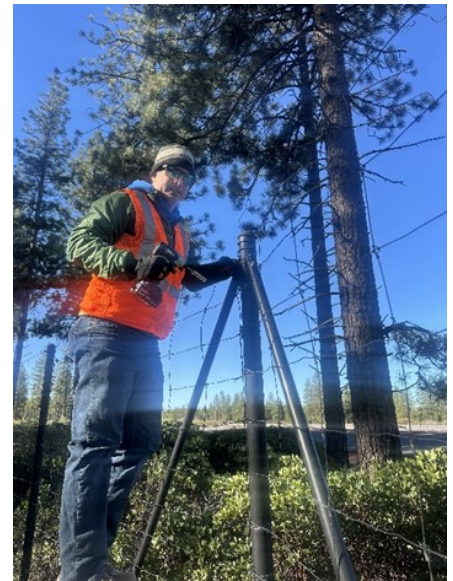
Brady is put to work tightening up an angle bracket.
