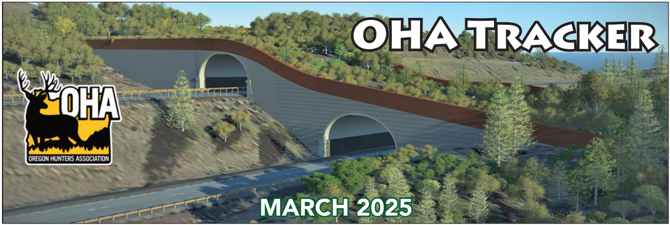
An artist's rendering shows the future wildlife crossing over Interstate 5 south of Ashland, which will be Oregon's first wildlife overpass. A similar new overpass in Idaho is already showing impressive results.
