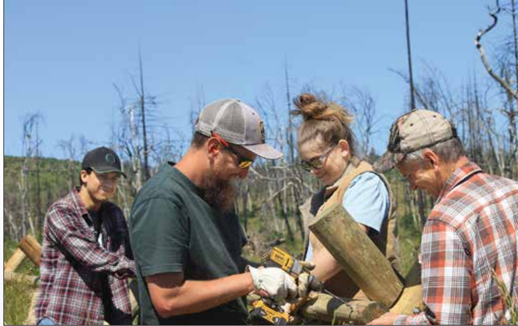
OHA volunteers helped construct nearly 4,000 feet of buck-and-pole fence to protect an aspen stand at the White River Wildlife Area on June 10 and 11.
