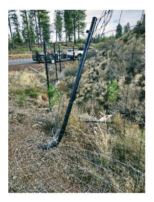
On the East fence at the very North end there were two locations on the fence that Elk have gone through and caused a lot of damage breaking wire, bending T posts and separating wire from the posts. We did the repairs.
