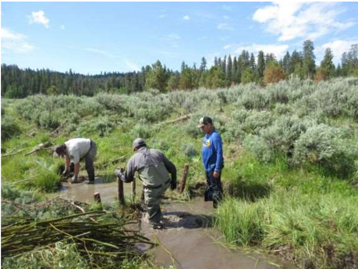
BDA being constructed
