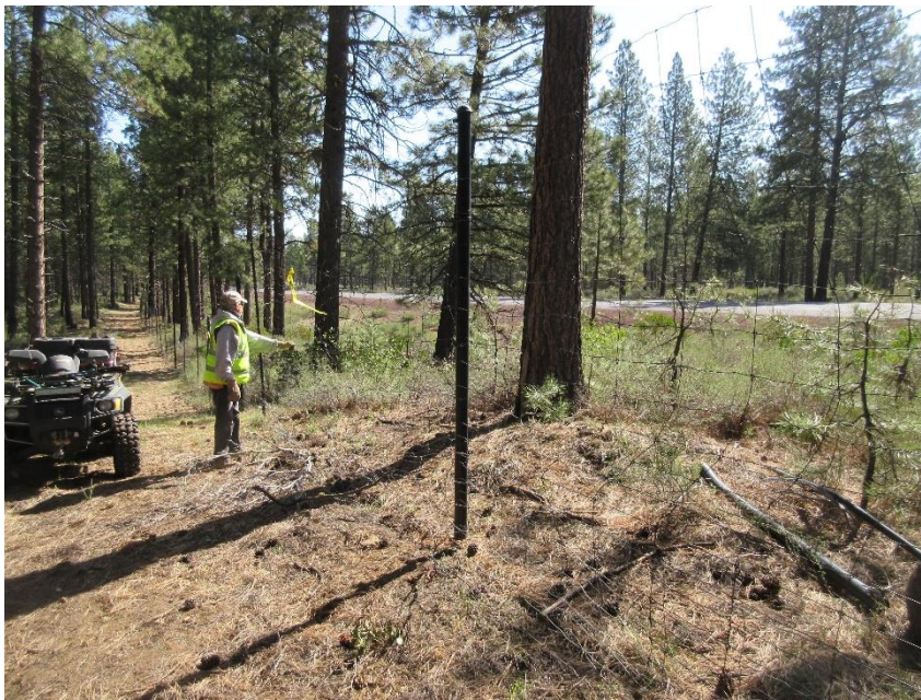
Steve Jones inspecting alcohol fueled fence damage done by an intoxicated motorist. Metal post and angle braces are in lower right corner of picture. Fence has been temporarily wired back together however a section of wire will need to be replaced along with the lower 3 foot wire which spreads out onto the ground.
