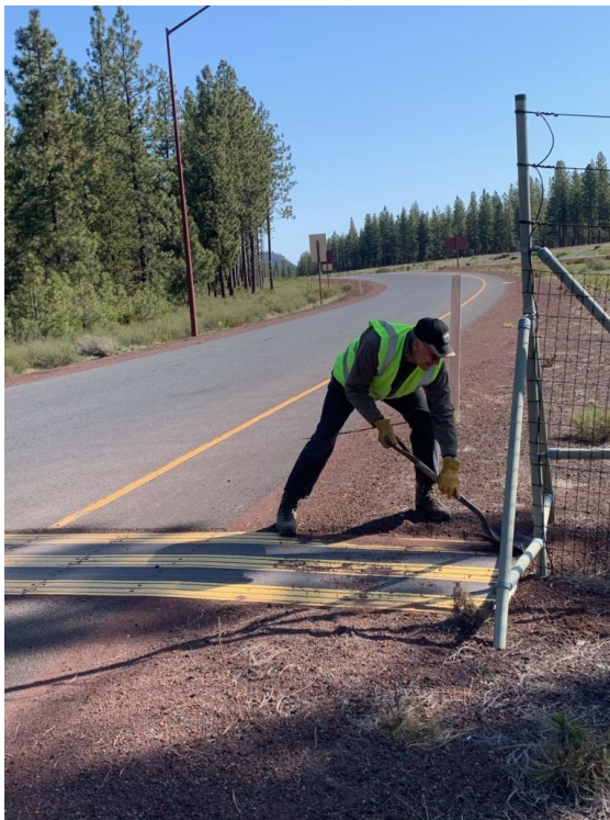
Greg Petsch left and Eric Brown right work on cleaning off the electric strips on the off ramps.
